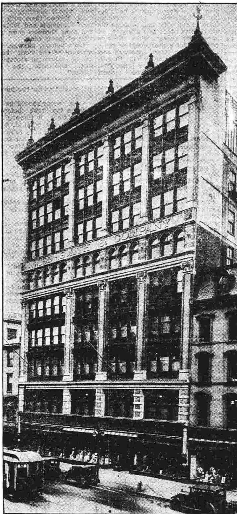
Five story structure (right) once site of old Roberts' Opera House, to be replaced by modern ten-story addition to Wise, Smith and Company.
